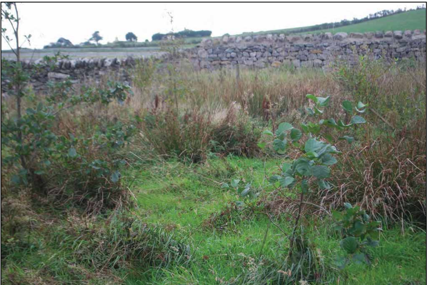
Plate 38 - Dalar Hir Farm and Fields area: Field 13, southern boundary - change in the wall styles indicating transition from an A5 boundary wall (left side) to an A55 replacement wall (right side)
